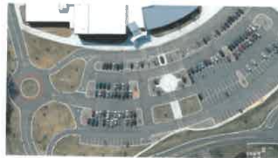
Pedestrian connections between rows of parking and the Walkertown High School.
