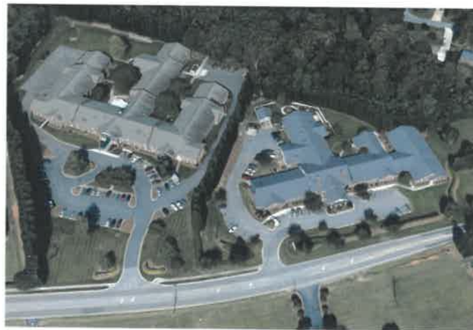
Robinwood Senior Living apartments located next to Kerner Ridge Assisted Living facility in Kernersville.
